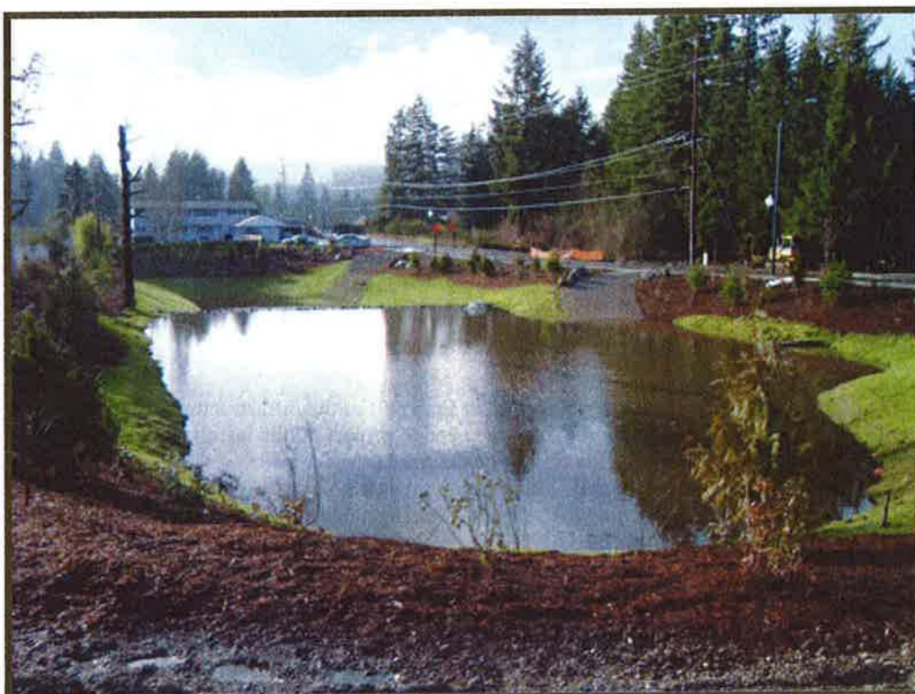
A stormwater pond captures and slows water runoff.
